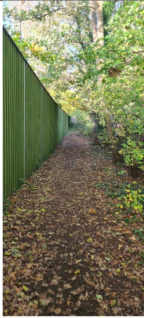
View of footpath to rear, showing timber fence alongside M25
